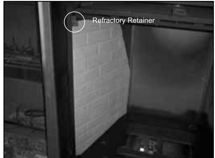
Figure 14.2 Install Left Side Refractory
